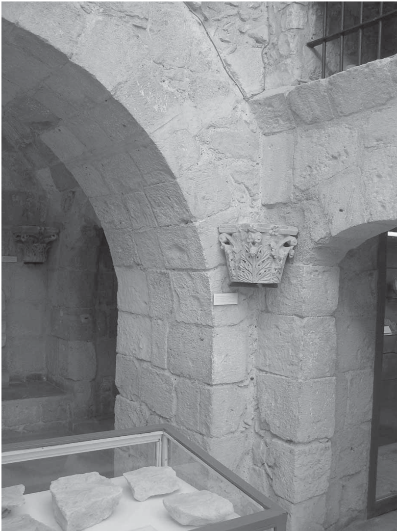
Fig. 52: Limassol Castle, upper level of cells, detail of south side of arch supporting the western wall of the eastern roof chambers [M. Olympios].
